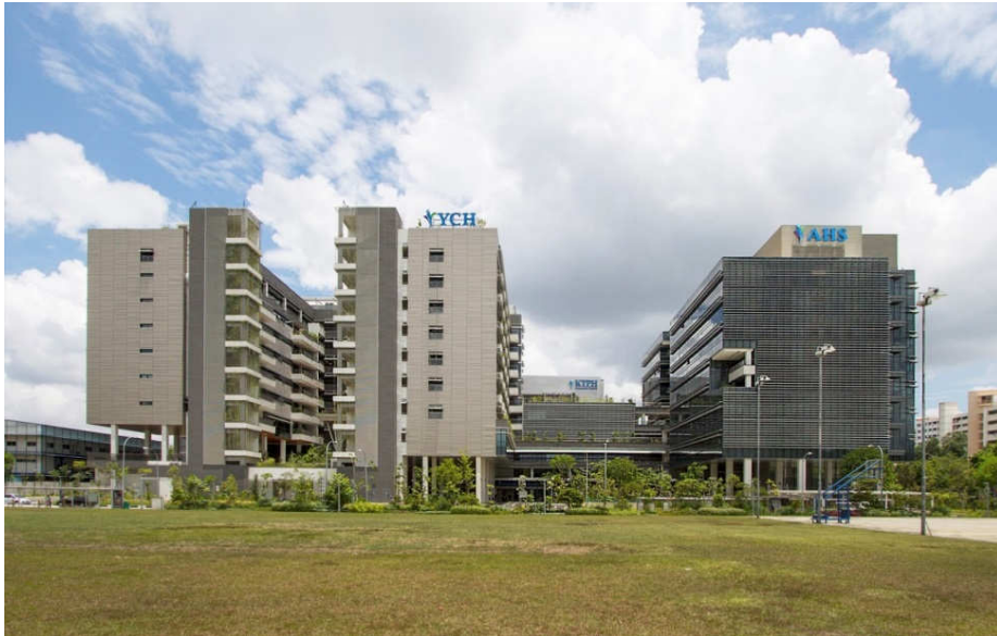
Yishun Community Hospital By Kimly – Shimizu Joint Venture
